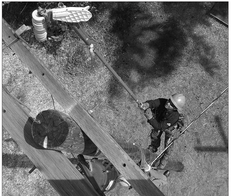
Clockwise from top left, Todd Niva lowers Joe to the groundmen waiting below; Bill Richardson gives the thumbs up to his groundmen after completing the pole-top rescue; Jeff Speelman reaches up with the hot stick to de-energize the cutout on the pole so he can safely rescue Joe; Groundmen Mike Purdy and Keith Lilly operate the hand line to the line-man, which is how they receive the hot stick as well as lower Joe.
