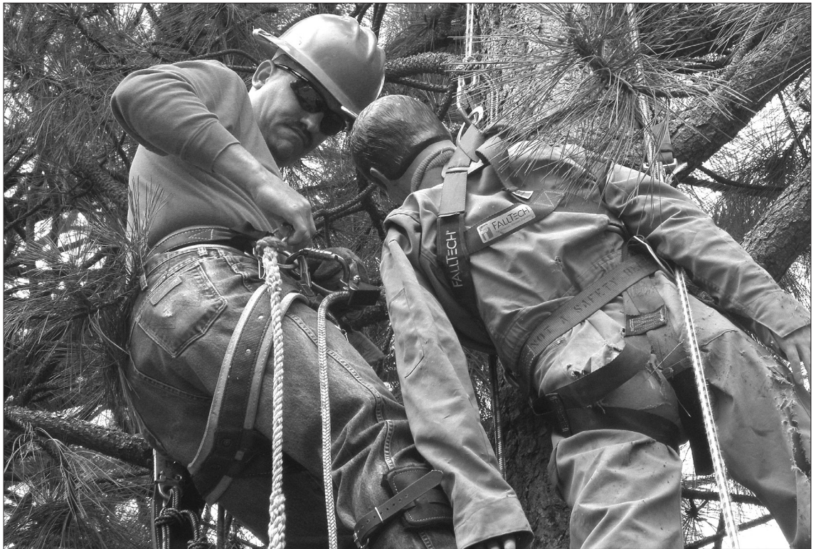
PUD employee Bobby Koffler prepares to perform a rescue drill at the top of a pine tree. His "victim" is Joe, a 180-pound dummy.
